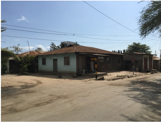
Picture 3. Typical detached home, Makumbusho, photo by the author
